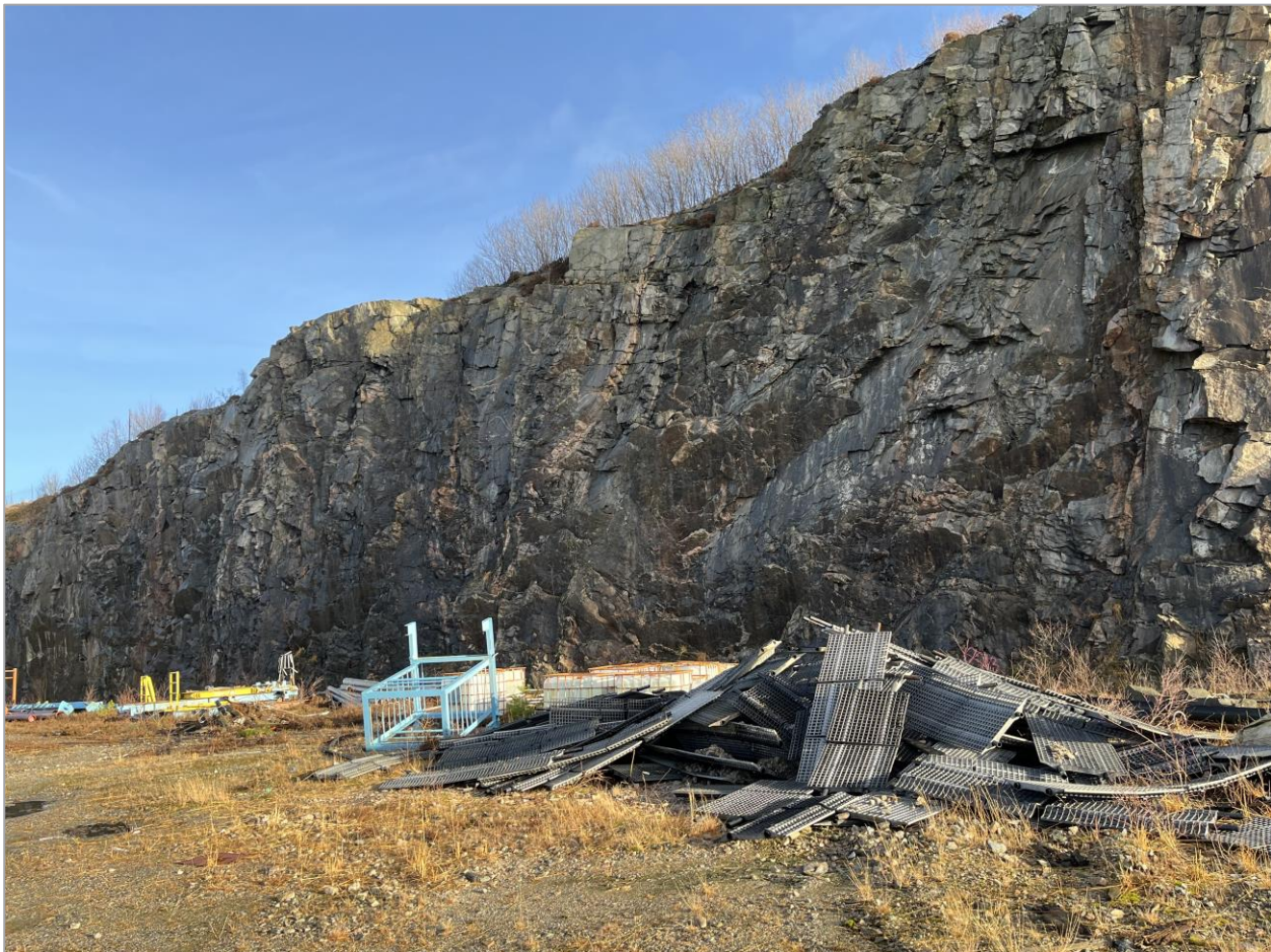
Figure 8 View of the large-scale rock wedge
