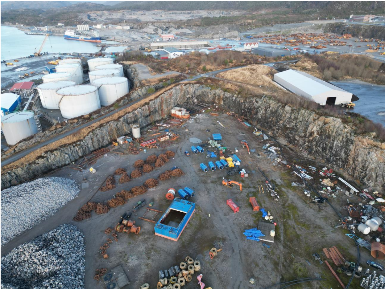
Figure 2 Drone photograph giving an overview of the site
